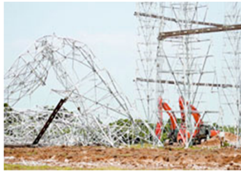
Demolition of the "Elephant Cage" Sobe Communication Site in 2007
